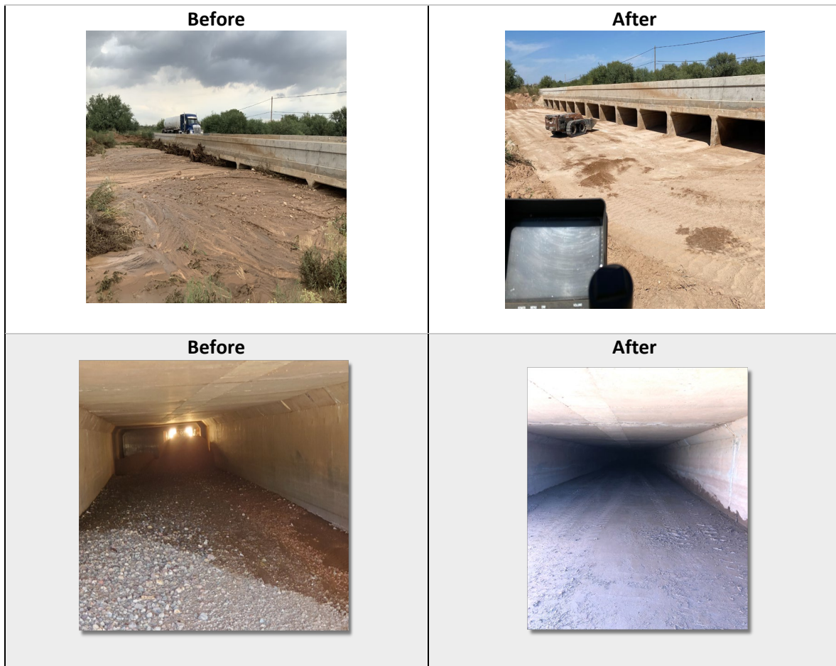
Figure 2. Remote-controlled Skid Steer and Clearing Effectiveness
